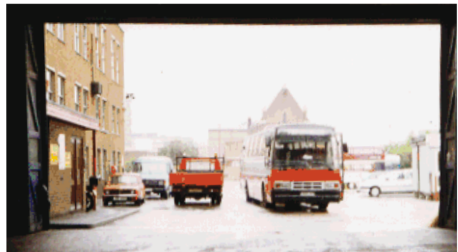
Figure 7 Bus garage with doors open so as to provide a steady flow of clean air
